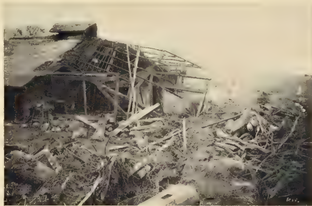
WRECKED BY AN EARTHQUAKE.
